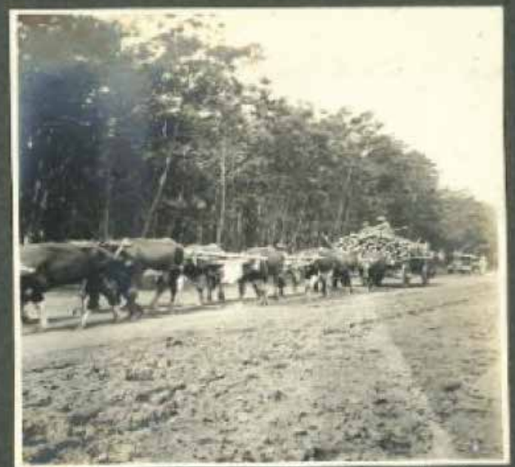
Bringing timber to rail
